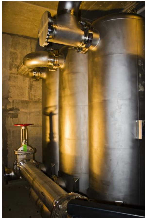
Fig. 2.4 – ^{16}N Delay Tanks in shielding vault
