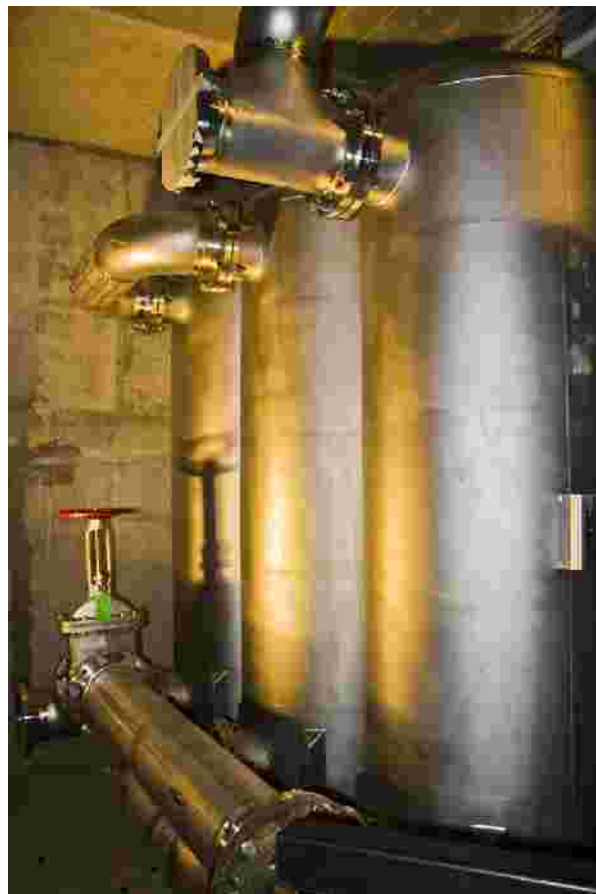
Fig. 2.4 – ^{16}\text{N} Delay Tanks in shielding vault
